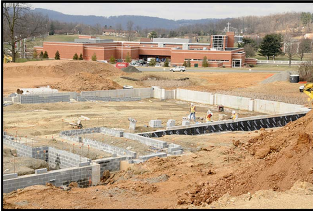
Figure 1: Footing Excavation and Constructed Foundation Walls
